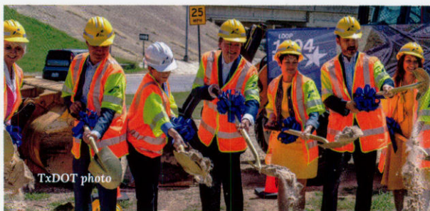
Texas Transportation Commission Chairman Bruce Bugg Jr. (fourth from left) kicked off construction on Segment 1 of the Loop 1604 North Expansion.
