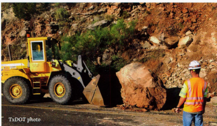
In mid-May, the Canyon Maintenance Section helped remove a rockslide that was blocking a roadway in Palo Duro Canyon State Park.
