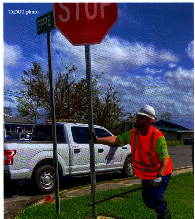
Lee Roy Bryan inspects a damaged sign in the aftermath of Hurricane Ida.
