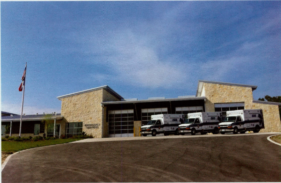
The new Bulverde-Spring Branch emergency services building opened in October. The 18,000 square-foot station has three ambulance bays and a fourth bay for a fire apparatus, classrooms, a library, an anatomy lab, sleeping quarters, crew kitchen—even a separate treatment room with a bed for walk-ins located just off the ambulance bays.
