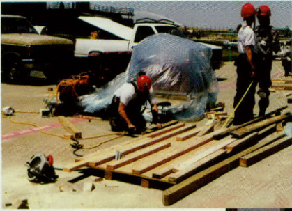
Above, after the Bonfire collapse, task force members had to devise strategies, including building shoring, to extricate the last two victims, who were located deep within the stack.
