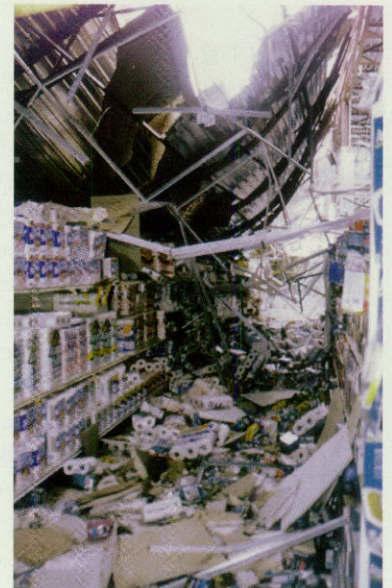
When an F2 tornado touched down in Cedar Park in 1997, rescuers called in the task force to help search the rubble of buildings, such as this Albertson's grocery store. Photo by Duane Smith courtesy of Hill Country News.
