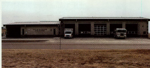
Plainview Fire/EMS opened a new station in February. With more than 10,000 square feet, the station has five engine bays and eight separate bedrooms for staff.
