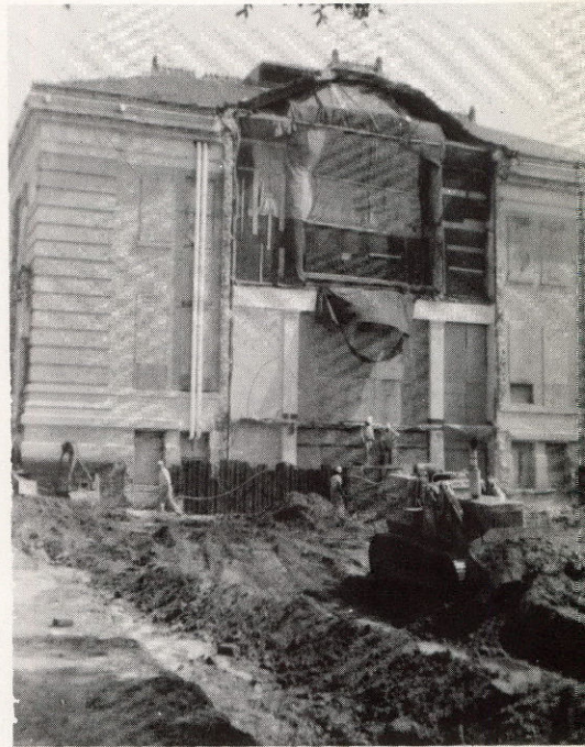
Construction at Rosenberg Library
