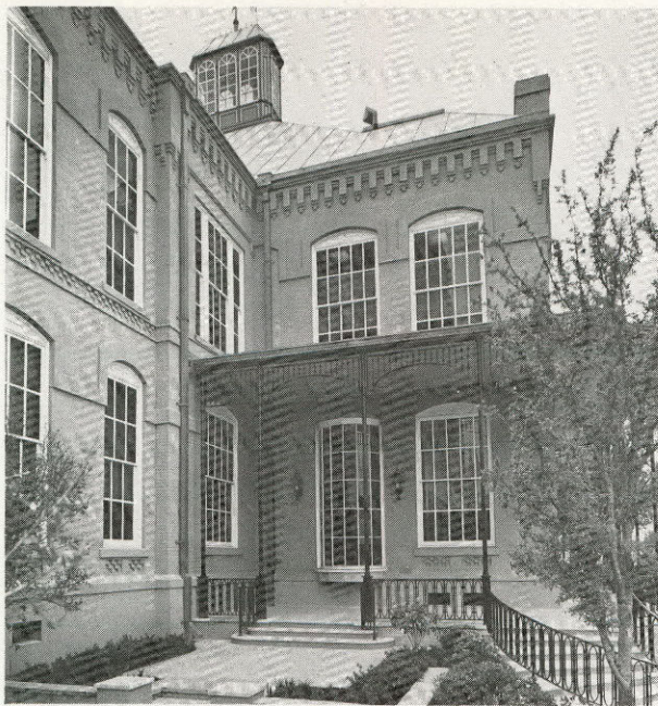
Views of Cumberland Hill School's Akard Street entrance before and after restoration show some of the changes that were necessary to restore the original architectural appearance.
