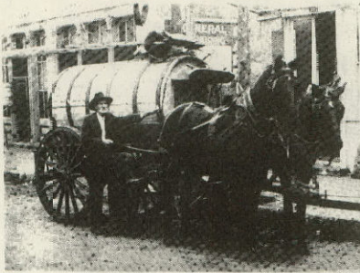
The water sprinkler
