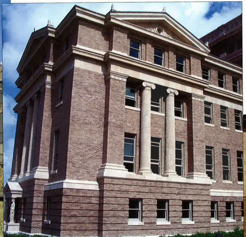
1914 Nueces County Courthouse
