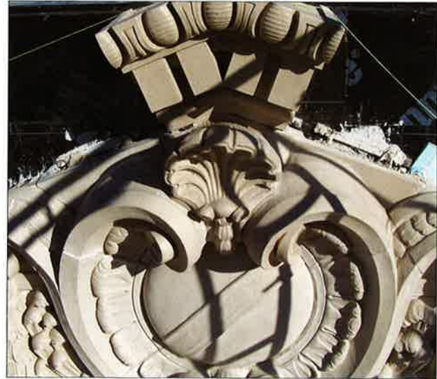
An 800-piece terra cotta jigsaw puzzle recreated the Williamson County Courthouse's original four ornamental porticos.
