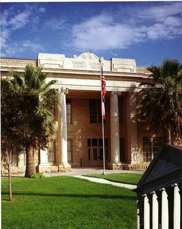
1926 Dimmit County Courthouse
