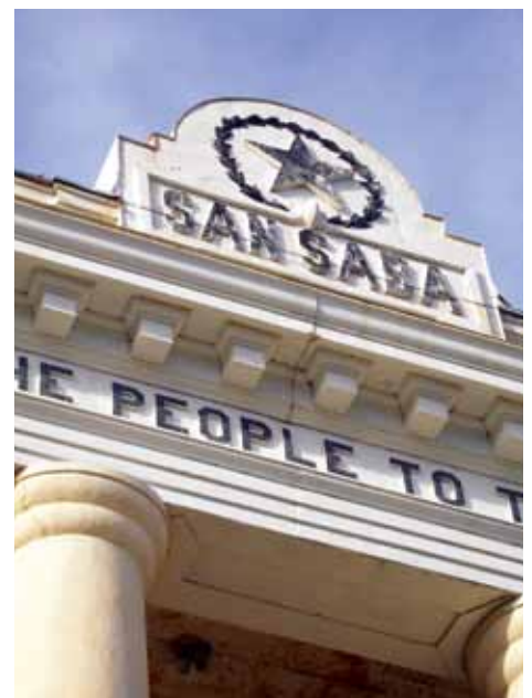
Right: 1911 San Saba County Courthouse, San Saba
