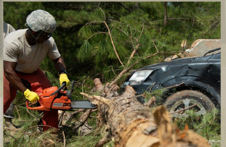
Air Guardsmen remove debris from a roadway during convoy training for a disaster area during state active duty missions. (U.S. Air National Guard photo by Staff Sgt. Emmanuel Gutierrez)
