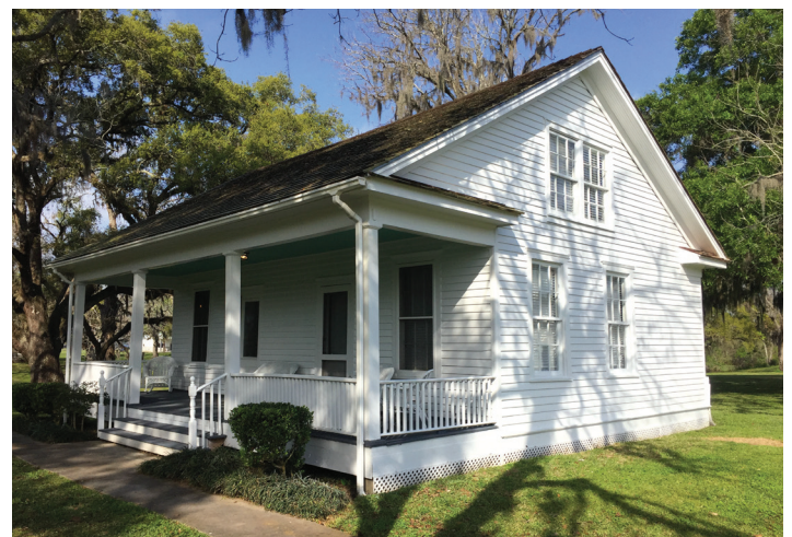
Top: Varner Creek threatened the Varner-Hogg Plantation. Above: The recently renovated Ranger's Cottage.
