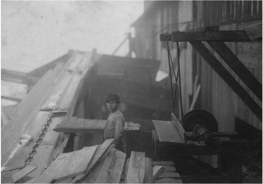
Fig. 4. "Dangerous work. Charlie McBride. Said twelve years old. This twelve year old boy has a steady job with the Miller & Vidor Lumber Company. He takes slabs out of a chute which has a moving endless chain to carry the wood up the chute. He passes the slabs onto the other boy who saws them on an unguarded circular saw. Charlie runs the saw himself whenever he gets the chance. He is exposed not only to the above danger, but to the weather—no roof even. Has been here for some months. 'Get four bits a day.' Fifty cents. Works ten hours. This was the only mill that I found around Beaumont that employed boys, likely because they are located some distance out of town. Location: Beaumont, Texas." See fig. 5 for note on Charles McBride. Courtesy of the Library of Congress (Rep. No. LC-DIG-nclc-04912)
