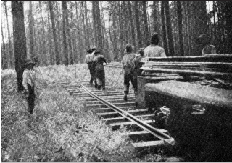
“Laying new tram road. Silsbee.” From John H. Kirby, Timber Resources of East Texas (1902). Courtesy of the Tyrrell Historical Library, Beaumont, TX.
