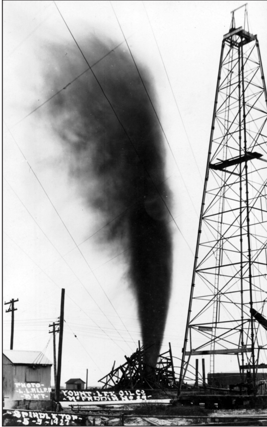
L. L. Allen, photographer. Blow out of Yount-Lee Oil Co. McFaddin No. 29 (1927). Courtesy of the Lamar University Archives and Special Collections, Beaumont, TX.
