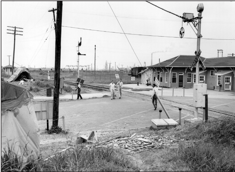
Picket line at the Main Gate on north end of Houston Street, April 29, 1950. Note the tents used as temporary shelter to the left. Courtesy of Elton N. Gish, Lumberton, TX.
