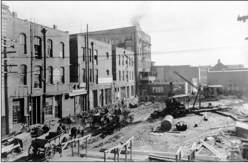
Construction of the Jefferson Theatre, Jan. 1, 1927. Courtesy of the Tyrrell Historical Library, Beaumont, TX.
