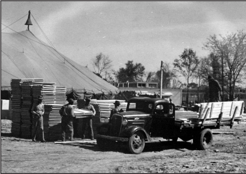
Workers loading prefabricated wood panels at the Multimax Village construction site, March 1942. Courtesy of the David Williams Papers, Edith Garland Dupré Library, University of Louisiana at Lafayette.
