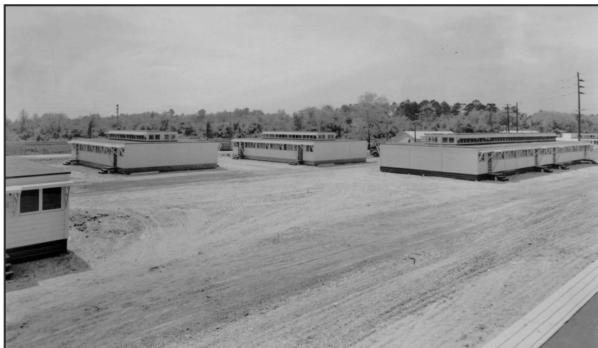
Housing modules at Multimax Village construction site, n.d.. Courtesy of the David Williams Papers, Edith Garland Dupré Library, University of Louisiana at Lafayette.
