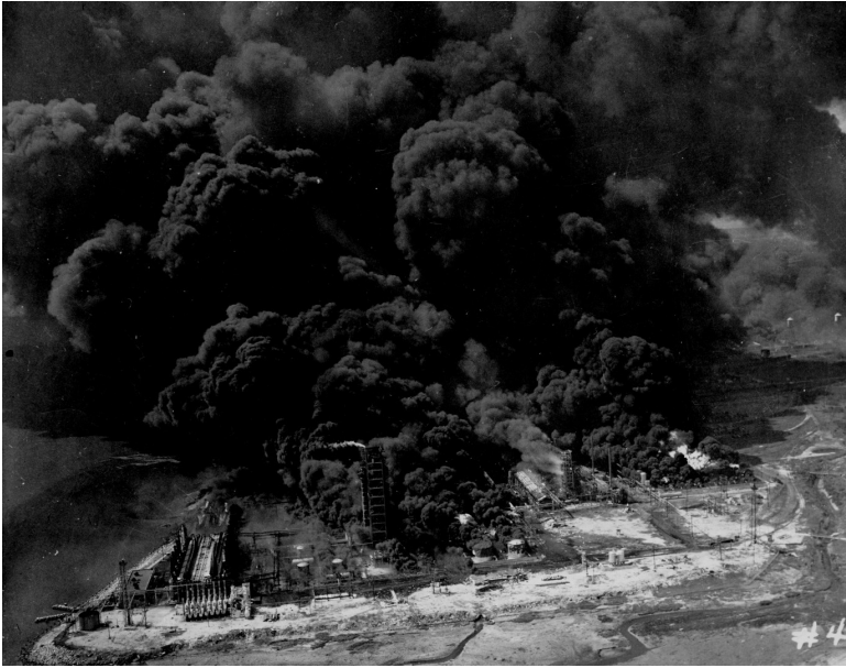
Monsanto Plant. Courtesy Moore Public Library, Texas City, TX.
