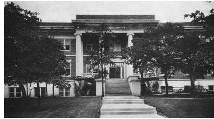
Brackenridge Hall, College of Industrial Arts, Denton, Texas
