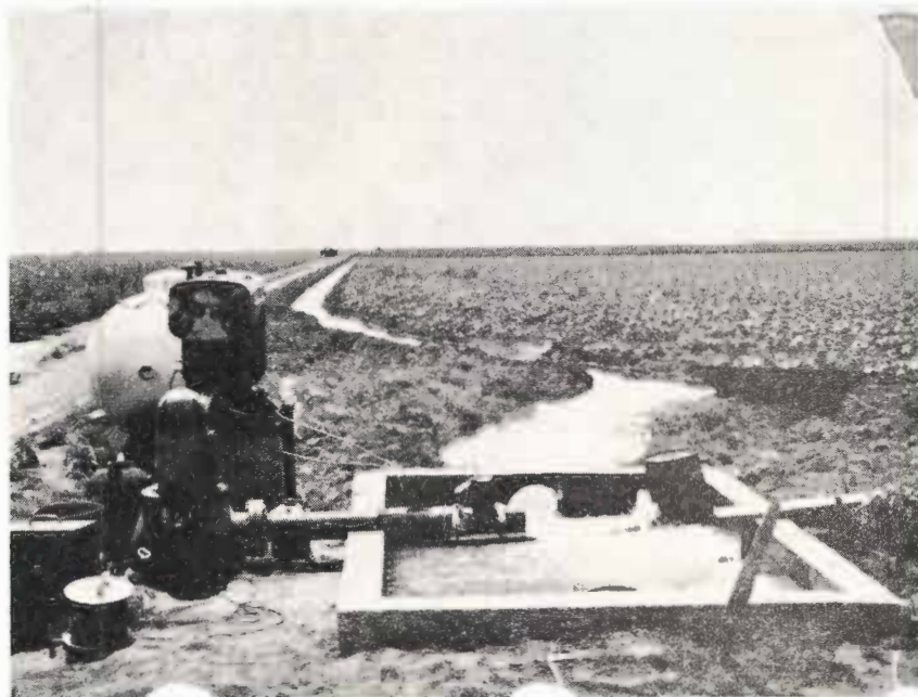
Well No. 2 on Joe D. Unfred farm. Note four-inch flow meter on discharge pipe and the open ditch in the background.
