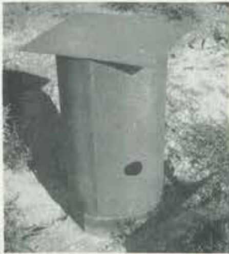
Pictured above is one method of properly closing an abandoned well.
