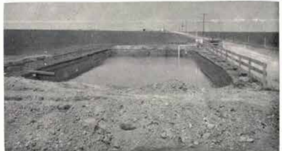
Picture shows "tail-water" being pumped from sump to higher land where it can be put to beneficial use.
