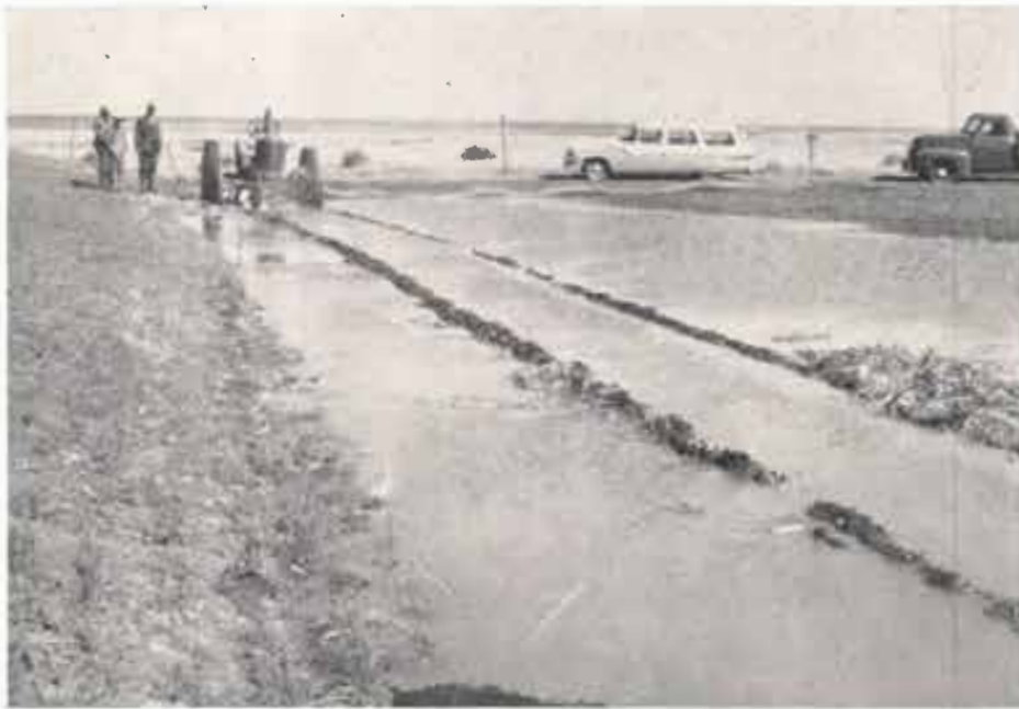
LOTS OF TAIL WATER — This photograph, made on the Wilbur Charles farm northwest of Bovina, illustrates a condition that is typical of many irrigated fields where the land slopes rather steeply.
