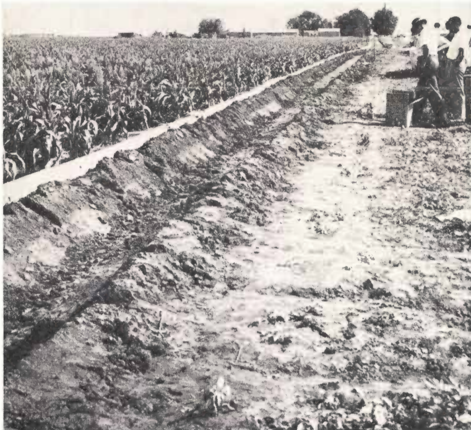
Flexible plastic pipe is used on the farm shown above to transport water from the well to the point where irrigation water is being applied. Closed systems are excellent conservation measures.
