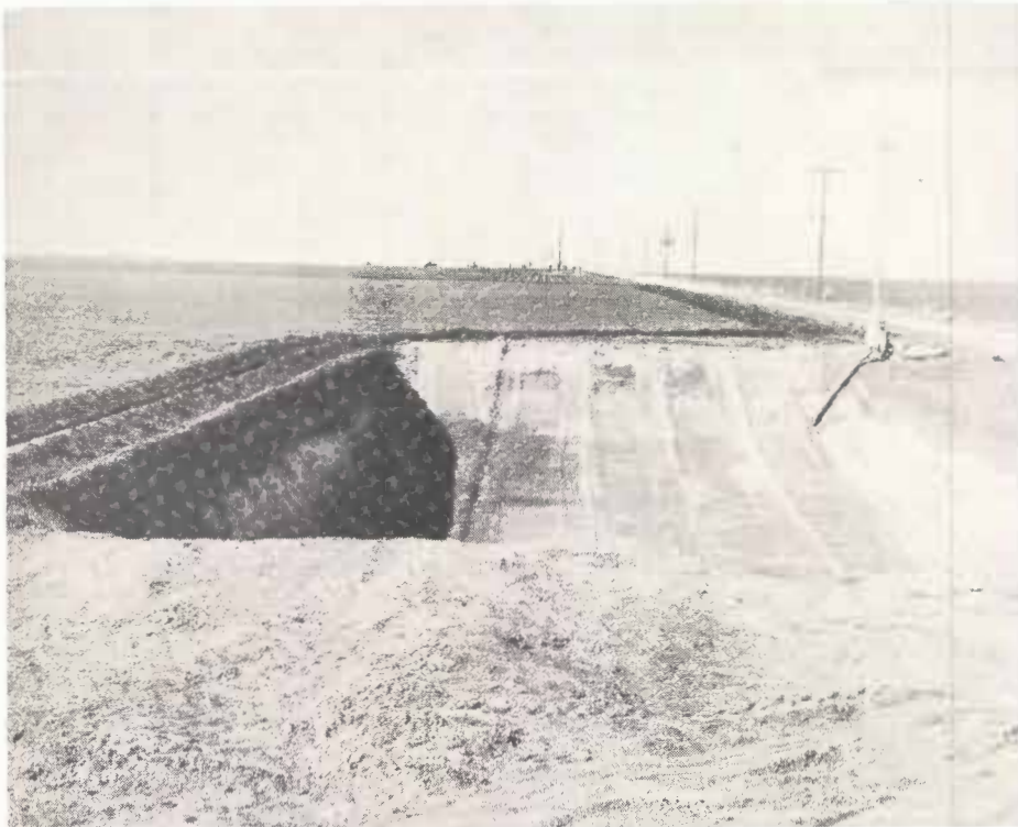
Sump 100 feet long x 40 feet wide x 10 feet deep was excavated to retain farm's "tail-water."
