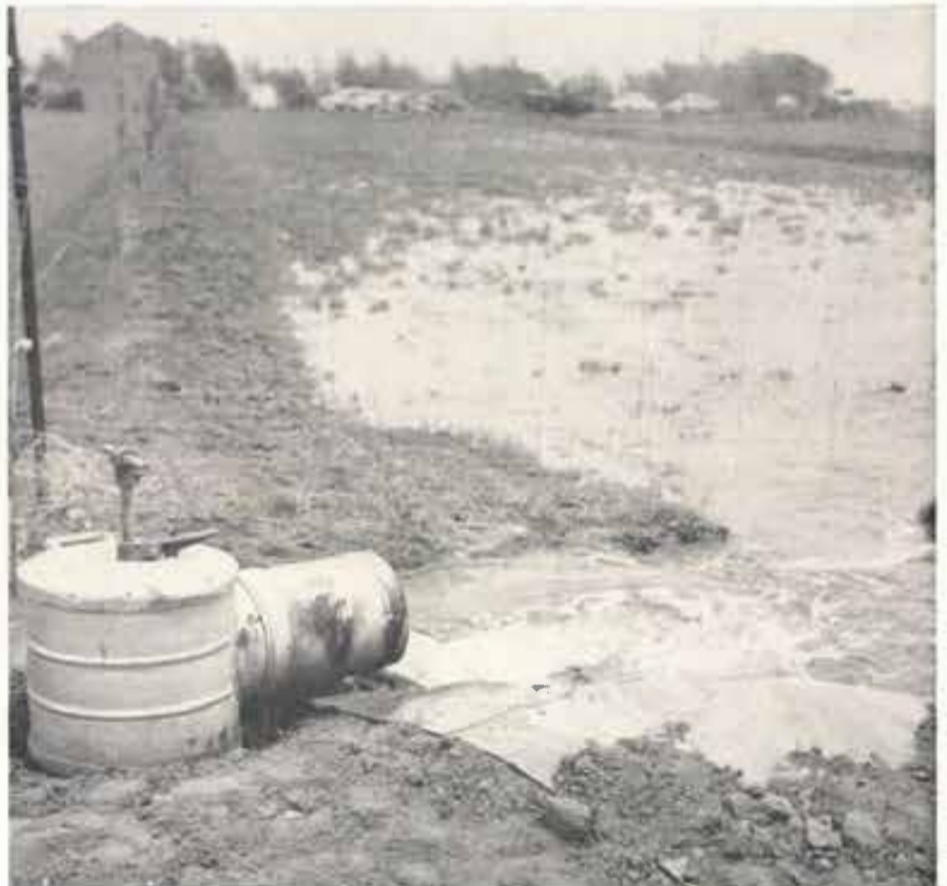
Underground concrete pipe has been installed on the above farm to conserve water. This type system saves water from evaporation and seepage, and it also affords the operator the convenience of plowing over the pipe.
