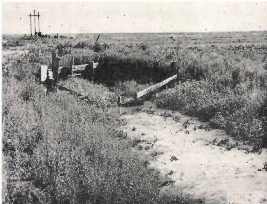
The above recharge well is 4 miles west of Hart and is on land owned by Willis Hawkins. From the lake the water drains through a dredged ditch to a 15-inch concrete well intake pipe. This pipe joins, at a gate valve, a 15-inch steel line coming from the well casing. The intake at the casing is 9 feet below the surface and is 1 foot below the lake bottom elevation. There are about 30 acres in this lake but not much water gathers in it because of the bench-levelled land which surrounds the lake.
