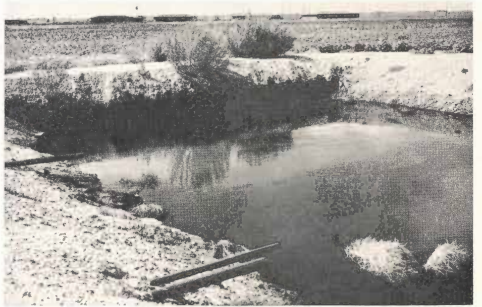
Pictured above is a surface salt-water disposal pit which is being used to dispose of oil-field brines on property owned by the Children's Home of Lubbock. This is a relatively new pit but in time the salt water which is put into it will probably percolate to the fresh underlying water. If this occurs, after awhile the concentration of salt will be such that the aquifer will become polluted.
