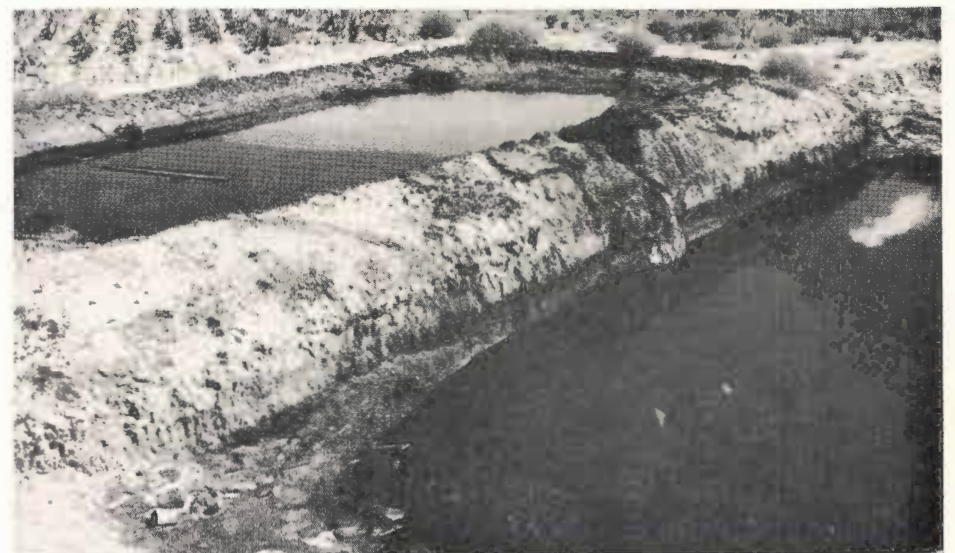
Pictured above is another surface salt-water disposal pit being used on the Children's Home farm. By using two pits side by side, the theory is that oil on the surface of one pit which is higher in elevation than the other will drain into the lower pit leaving only salt water in the upper pit. This plan supposedly facilitates evaporation by draining off the oil slick which is usually present. It may be noted in the picture that about half the upper pit is still covered by an oil slick.
