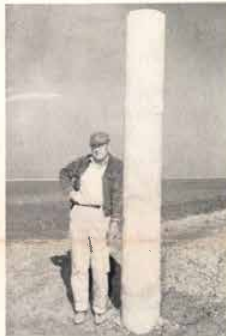
Lindsey L. Dycus stands beside an air-vent riser, which is part of his underground pipeline.
