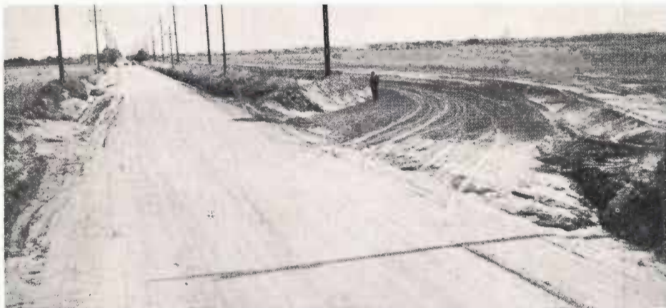
Pictured at left is shown the inlet to the main diversion ditch. The picture was made looking east down Erskine Road from the intersection of Erskine and Quaker. You will note the dam in each bar-ditch to divert water onto the farm from the road.
