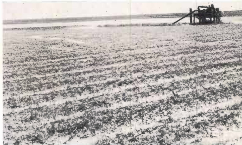
Another recharge project is shown above. This installation is on land owned by E. C. Jones and is 1 1/2 miles east of Olton. On the platform, which is about 8-feet high is mounted a 6-inch centrifugal pump, engine and fuel tank. When the lake catches water the pump is started and the water transported to either an 8-inch well approximately 500 yards away, through underground pipe, or put on the benched land which surrounds the lake.
