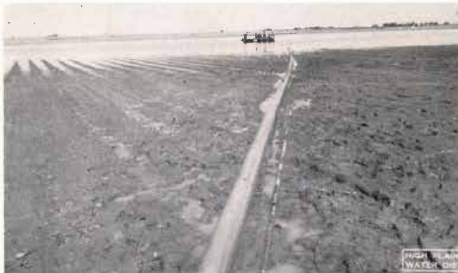
This year Mr. E. W. McFarling, who has a permanent recharge installation on his home farm, excavated a hole 8 feet deep, 30 feet wide and 200 feet long in the bottom of a lake on another of his farms 4 miles west of Lubbock. With dirt dug from the hole, Mr. McFarling levelled the bottom of the lake so all water would drain to the hole. The lake was filled by rain. During June, a 2200 lb. trailer was floated at the hole in the lake by 14—55 gallon oil drums. On the trailer is mounted a 4-inch centrifugal pump and engine. The pump delivers lake water to an 8-inch irrigation well. The lake water is discharged into a concrete riser and from there it goes into the pump discharge pipe and into the well. Mr. McFarling rented 440 yards of 2-inch gas line to carry fuel from the irrigation well engine to the centrifugal pump engine.
