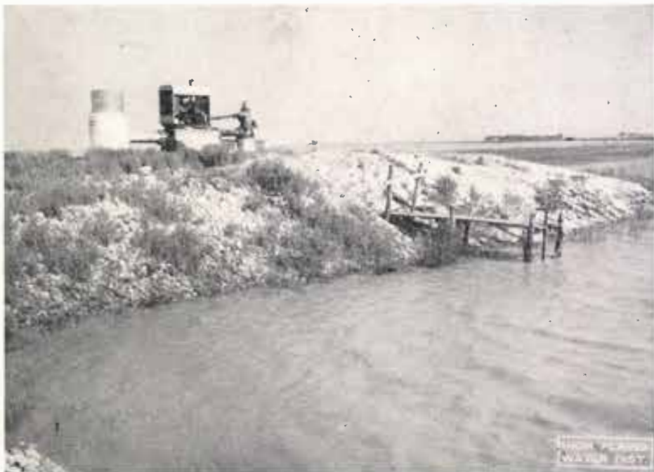
Pictured above is a permanent combination recharge and production well located on a farm 4 miles west of Lubbock and owned by E. W. McFarling. The lake pictured covers about 20 acres and on June 4 the lake contained approximately 40 acre-feet of water (estimated by W. L. Broadhurst). On June 14 the lake was completely drained into the recharge well. The well is pumped twice each day for 15 minutes in order to clear the well formation of lake mud and silt. The well was drilled 5 years ago to a depth of 190 feet. The recharge part of this installation was constructed at that time and the well has been used since for recharge as well as production. An 8-inch steel pipe carries the lake water to the casing by gravity flow through a gate-valve.
