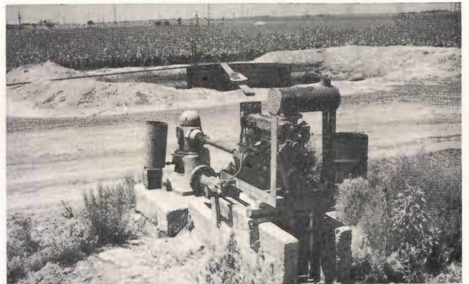
Picture above, in the foreground, is Irrigation Well No. 2, which is located on the illustrated farm plat. In the background can be seen a surface salt-water disposal pit which is on the property that adjoins the west line of the Children's Home. The irrigation well was abandoned in July 1957 because of salt-water pollution.
