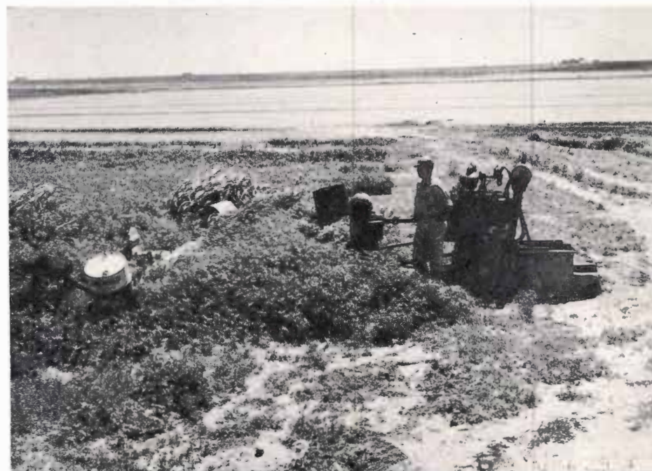
Another recharge project is shown above. This installation is on land owned by E. C. Jones and is 1 1/2 miles east of Olton. On the platform, which is about 8-feet high is mounted a 6-inch centrifugal pump, engine and fuel tank. When the lake catches water the pump is started and the water transported to either an 8-inch well approximately 500 yards away, through underground pipe, or put on the benched land which surrounds the lake.
