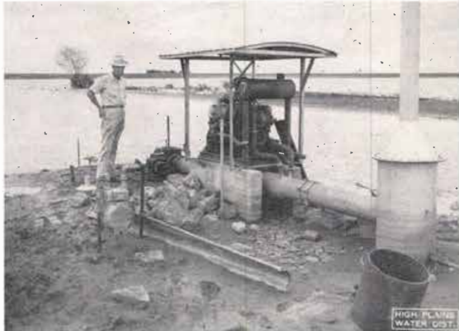
Pictured above is a recharge well on a farm located 3 miles north and 8 miles west of Lubbock which is owned by Russell Bean. Mr. Bean is shown in the picture. The well is at the edge of a 20-acre lake which averages about two feet in depth when filled normally. The lake has been completely drained three times this year and at this time is being drained for the fourth time. The well is pumped twice each day for a period of thirty minutes. Recharge intake extends 350 feet to the deepest part of the lake. Lake water flows into the casing by gravity.
