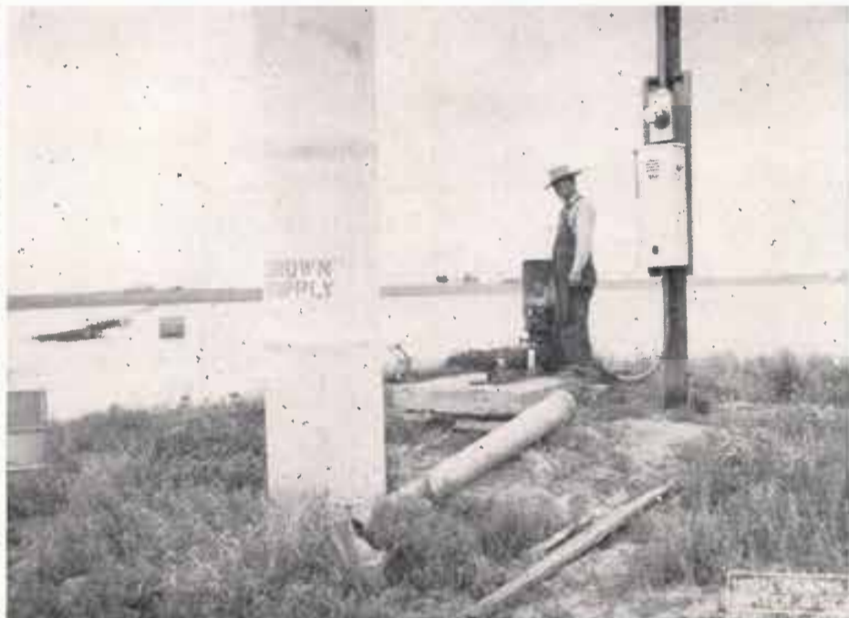
The recharge well shown above is on a farm owned by P. J. James, 4 miles east and 1 mile north of Shallowater. Medford Melton, farm operator, is shown at the well. The lake covers approximately 45 acres; however, 15 acres of it are on the adjoining land. Before May 1 the recharging began and has not been stopped since. The lake has been drained into the well almost completely 4 times, and at the time this picture was taken (June 17) the lake was full again. Pump is started each 12 hours and operated for 20 minutes to pump out silt. An 18-inch concrete line carries the lake water to the well casing where it drains in by gravity. This lake catches run-off water from about 3 square miles, and contains more water than can be handled adequately with only the one well.
