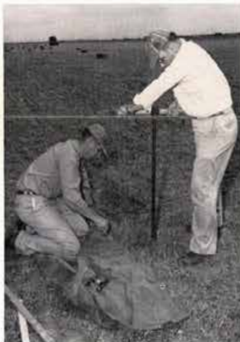
The pictures above show the steps which are followed to install meter blocks. (1) A small hole into which
