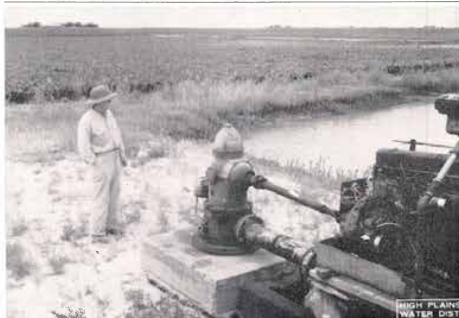
E. W. McFarling, who farms 5 miles west of downtown Lubbock, operates a combination recharge and production well. He has dug a large pit near the well at the low side of a wet-weather lake so water that collects in the lake will drain toward the pit. The recent rains filled the pit and lake, backing water up over about 5 acres of grain sorghum that was planted in early May. When the rains subsided, Mr. McFarling commenced to recharge the water into his combination well. In 5 days and nights all the water standing on the grain sorghum was gone and only a small amount of water still remained in the pit. The picture above shows Mr. McFarling surveying the grain sorghum that would probably have been lost had it not been for the recharge well. He also salvaged a considerable amount of water that largely would have been lost into the atmosphere through evaporation.
