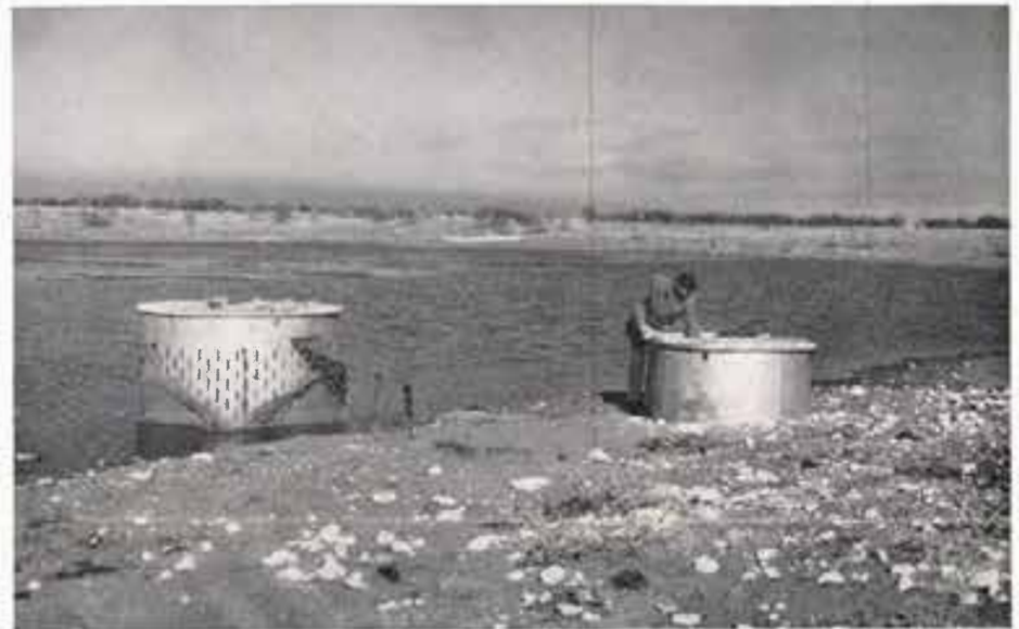
John Havens, U.S.G.S. geologist at Lovington, inspects a recharge well at the edge of a wet-weather lake in the Lea County Underground Water Basin. The large metal tank in the water, shown at left, is a filter made of a 6-foot diameter cylinder inside an 8-foot diameter cylinder. The space between the two cylinders is filled with pea-size gravel. The lake water gravity flows through the filter into the recharge well and ultimately out into the underground formation.
