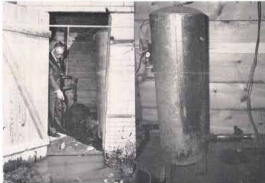
In picture at left above, W. R. Bradford, Lubbock City-County Sanitation Officer points to probable source of trouble for this contaminated domestic well. Surface water from rainfall drains toward the well carrying debris and waste into the well. At right, is shown a well properly constructed—the casing is extended above the well platform and concrete run between the well wall and casing from the water level to the surface. No surface water can enter the well.
