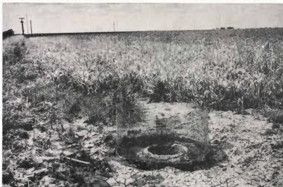
The picture above shows the intake of the recirculating system. It is located at the low end of the field so that all "tailwater" flows to it by gravity. The wire around the intake keeps out trash and stalks.
