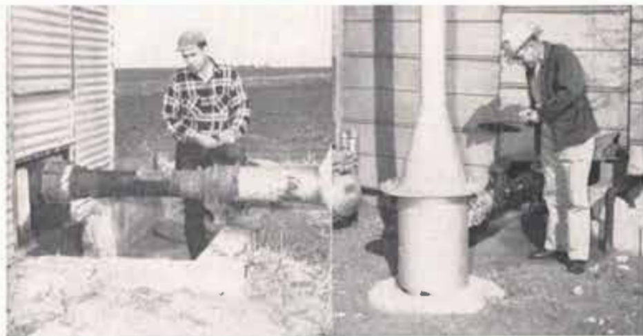
Buddy Winters, left, and Grice Herrington, Lubbock County farmers, are shown reading flow-meters installed on their irrigation wells to record amounts of underground water pumped to alternate-furrow test areas on their farms.
