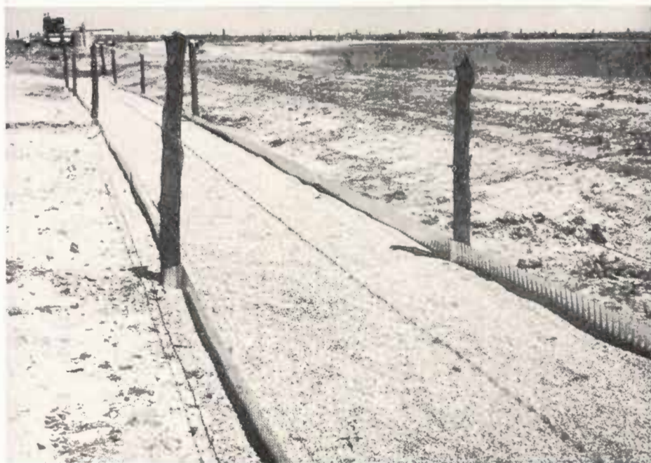
Figure 5 A layer of pea gravel about 30 inches thick, was placed in the trench from just above the shutter screen to ground surface. The pea gravel is designed to filter the lake water.
