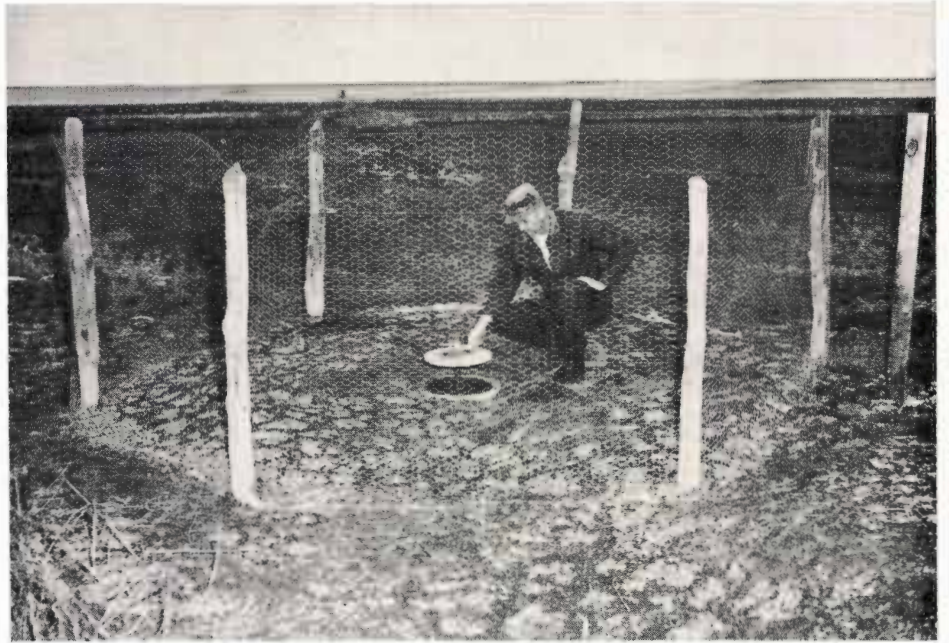
August Falkenburg, Estacado farmer, is shown adjusting the intake valve of the lake-pump system installed on the L. B. Cooper farm this past Spring. The intake was located in the deepest part of the wet-weather lake so that all the water would gravity flow to it. The wire fence installed around the intake is placed there to keep trash from entering the pipeline. In the background, near the center, the lake pump can be seen.
