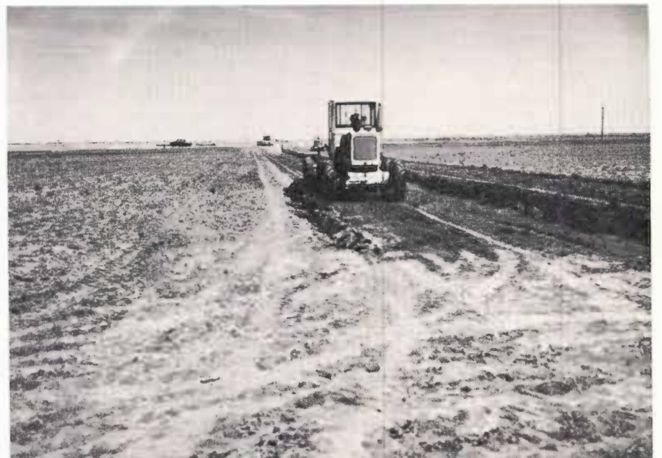
Figure 2 Maintainer prepares a channel in the bottom of the wet-weather lake. The channel is the lowest part of the lake; consequently all water drains toward it.
