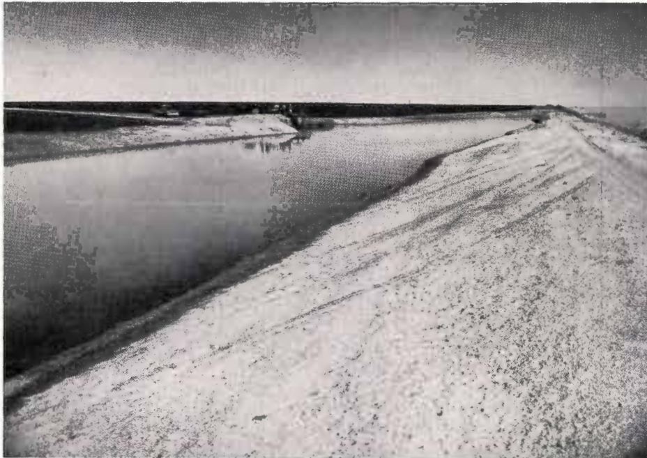
Dirt removed in constructing the "tailwater" reservoir was used to build the large earth dam shown in the foreground. Irrigation "tailwater" from 960 acres of Carnahan land runs into the reservoir where the centrifugal pump is shown in the background pumps it back to the top-side of the farm where it is used. The Carnahans state that the recirculating system not only saves irrigation water that was previously lost but that it is also better than having another good 8-inch well. The cost of pumping the water is much less than producing the same amount of water from the underground supply.
