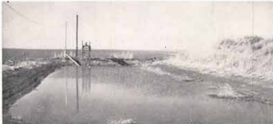
The picture above shows one of J. G. Evans' pump-back pits in Deaf Smith County. Irrigation "tailwater" gravity flows into the sump where it is picked up by a centrifugal pump and sent back to the high side of the farm through an underground pipeline. The water is thereby put to beneficial use rather than being lost by allowing it to meander to a nearby dry lake via road bar ditches as it once did.
