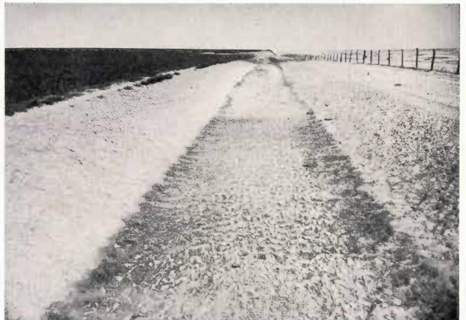
Large waterways have been excavated along the bottom of the fields to carry "tailwater" to the reservoir.
