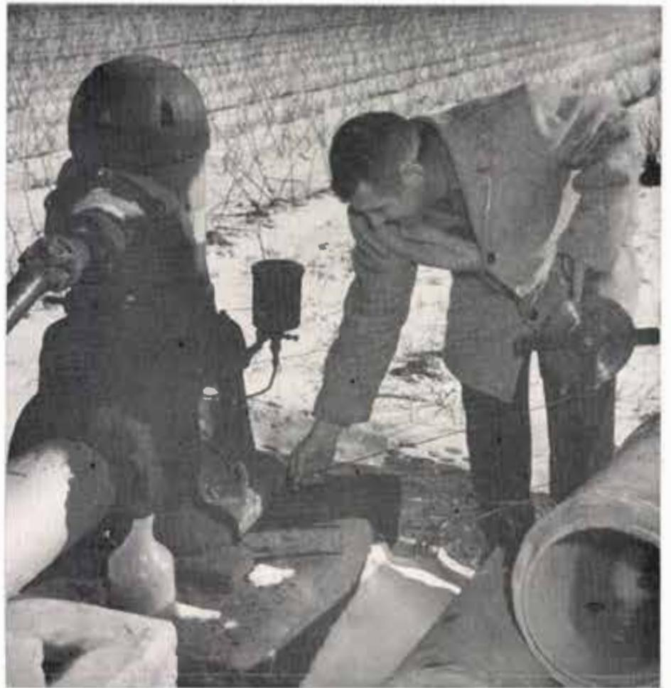
Wayne Wyatt, field representative for the Water District, is measuring an observation well. In this picture the graduated, steel tape is being inserted into the well annulus. After the well has been measured, a loose tag will be attached, which will have the 1963 and 1964 measurements on it.
