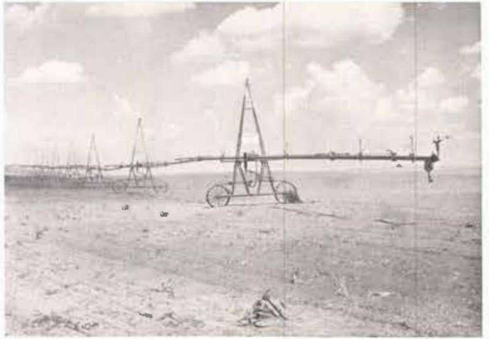
The self-propelled sprinkler system moves in a straight line around a pivot point at the center of the square-shaped farm.
