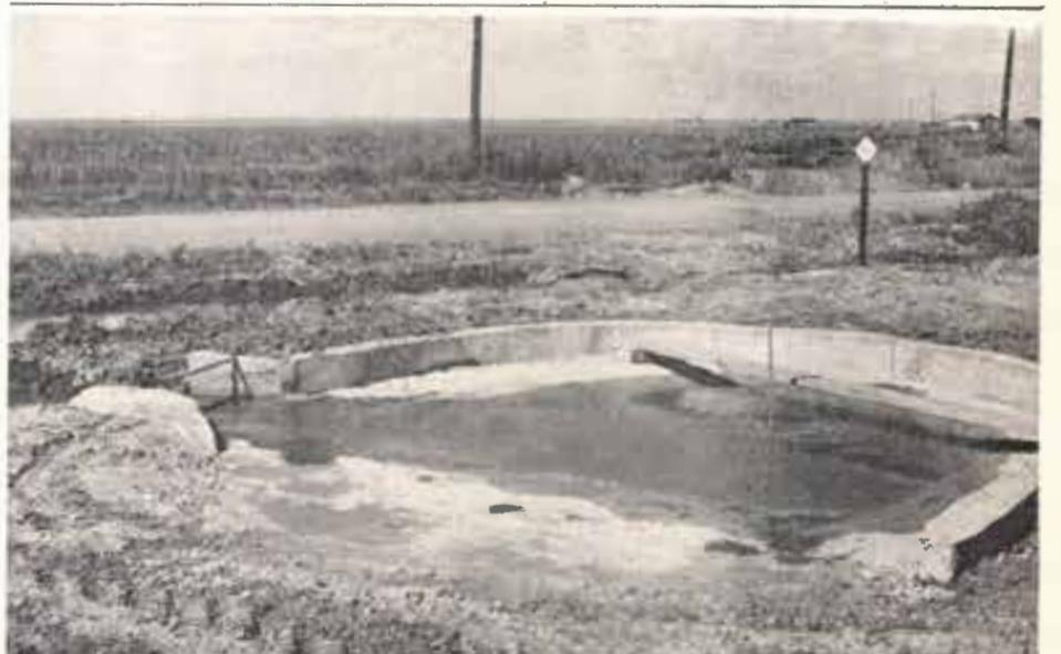
at left the portable dam installed in the road bar-ditch to divert "tailwater" into the sump. Picture at right shows "tailwater" in the sump as it enters the pipeline that conveys it under the road and into an irrigation "headwater" ditch from where it is syphoned onto a milo field.
