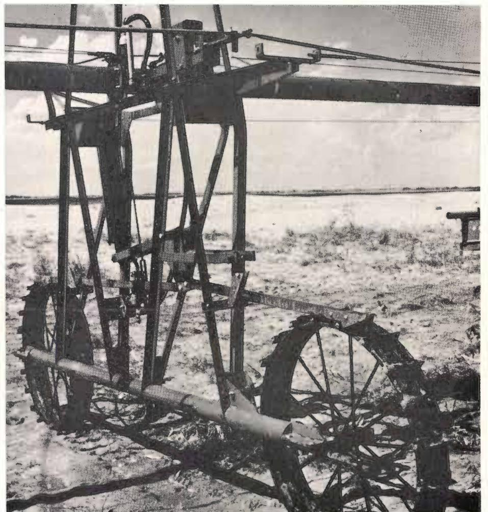
Note manner in which the horizontal bar engages with the wheel lugs when the cylinder is emptied. It is now prepared to slowly move the tower, and thus the pipeline, as the cylinder fills with water.
