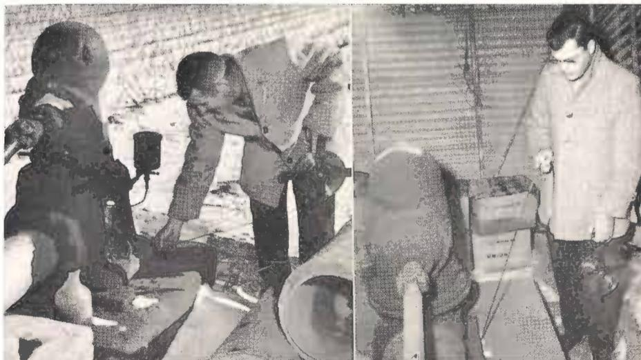
Wayne Wyatt, left, and Don Reddell, members of the High Plains Water District staff, are shown above as they measure the depth to water in two observation wells. Through this program, the fluctuations in ground-water level from one year to the next are determined. At a later date, water level measurements will be published in "The Cross Section".
