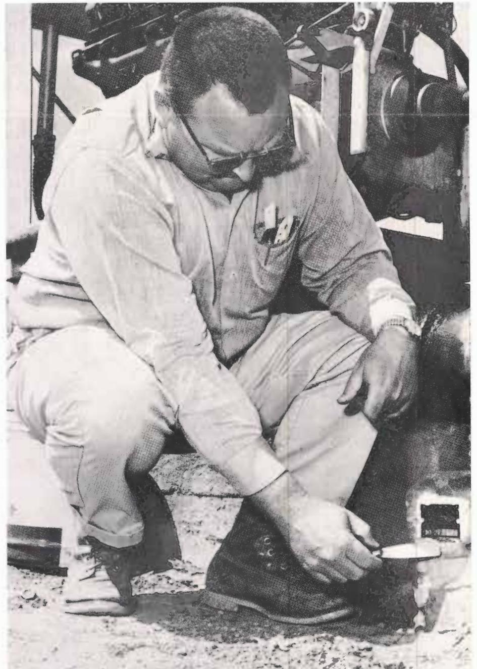
Frank Rayner, Texas Water Commission, is placing an identification tag on the concrete base of a pump. The tag, and the number stamped on it are used for identification.
