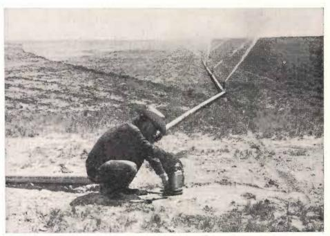
When the lateral line is in position for the next setting all that remains is attaching it to the main line and opening the valve which allows water to flow through to the sprinkler outlets. Shofner can change settings of his two one-quarter-mile long laterals in about 30-minutes.
