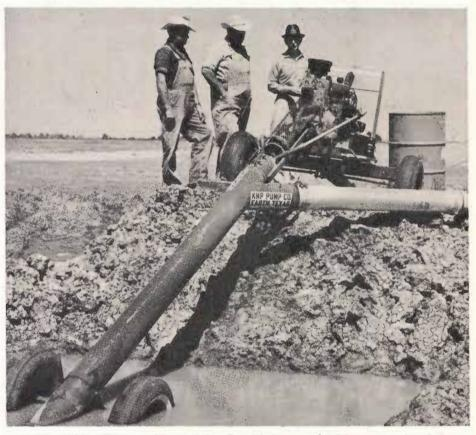
Charles White, Ernest White and Gus Parrish inspect the lake pump after it has been placed on the dump. This will be the permanent location for the pump, as it is above the high water level of the lake. Because the pump's bowls are submerged, it needs no priming.
