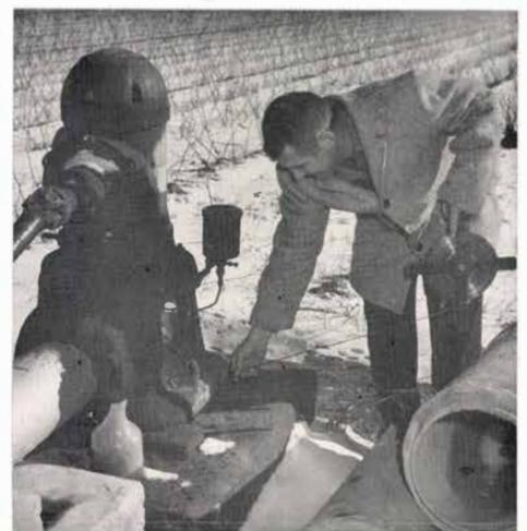
Wayne Wyatt, field representative for the Water District, is measuring an observation well. In this picture the graduated, steel tape is being inserted into the well annulus. After the well has been measured, a loose tag will be attached, which will have the 1963 and 1964 measurements on it.
