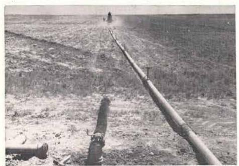
Each change in setting means moving the total length of lateral line across the main line to the opposite end of the tract to a new position 50 feet farther along the main line. The tractor is angled slightly away from the wetted area to accomplish each move. It naturally takes some practice, but in a short period of time the tractor operator learns the proper path to travel in order to position the line for the next setting.
