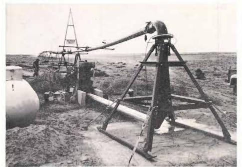
The pivot is guyed from a concrete base. Nix' well, shown left of center in the photograph, produces about 700 g. p. m. at 70 p. s. i. In length the system reaches from the center of the farm to the nearest property line 440 yards away.
