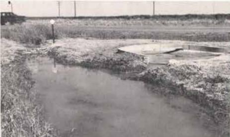
Above is shown a sketch of the G. D. Anderson farm near Friona. It indicates the relative location of the concrete sump installed on the farm to salvage irrigation "tailwater" that in the past was not beneficially used. Note in the picture
