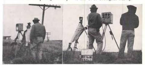
Pictured above are Yukio Yamamoto and Charlie Lough with the U. S. Geological Survey. They are shown using some of the modern surveying equipment, high-precision theodolite, electronic transit, high-frequency transceiver, and mobile elevation meter, employed to obtain field data for use in making topographic maps within the High Plains Water District. (Photo—Texas Water Commission)
