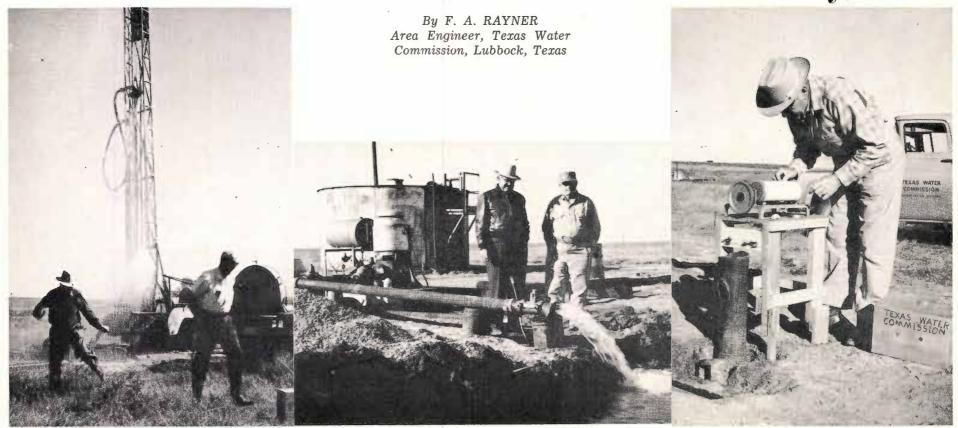
T. B. Duggan, Cochran County farmer-rancher and F. G. Courtney with the Gulf Oil Corporation, are shown in the photograph at left as they hurry to escape the spray of water being blown by compressed air from a test well drilled into the Cretaceous sands on land owned by Duggan located south of Whiteface in Cochran County. At center, Duggan and a friend watch as water is pumped from the Cre-
