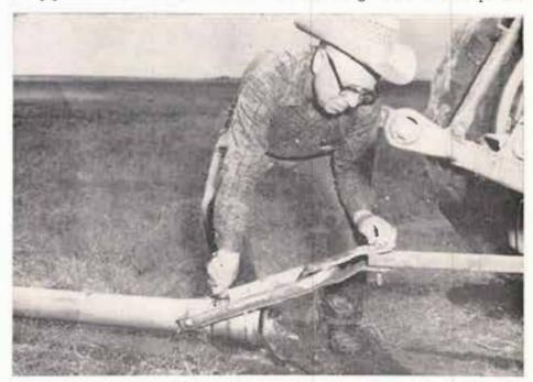
When Shofner changes the setting of his latural lines, first the water supply is cut off, the line disconnected from the main line and allowed to drain. Then the lateral is attached to the tow-bar of his tractor for movement to the next setting.
