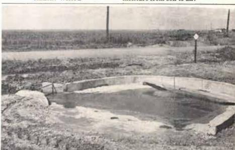
at left the portable dam installed in the road bar-ditch to divert "tailwater" into the sump. Picture at right shows "tailwater" in the sump as it enters the pipeline that conveys it under the road and into an irrigation "headwater" ditch from where it is syphoned onto a milo field.
