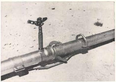
The tow-move coupler is relatively simple and serves to hold two ordinary lengths of sprinkler pipe together. To facilitate its movement along the surface of the land, the bottom of the coupler is built in the form of a skid. The coupler has a pin in the center of the skid to allow slight lateral movement.
