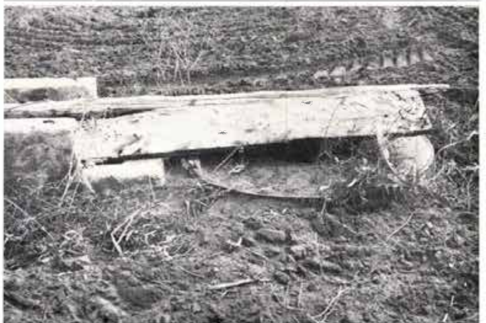
Abandoned wells like the ones pictured are hazards that can and will cost a life if not properly closed.
