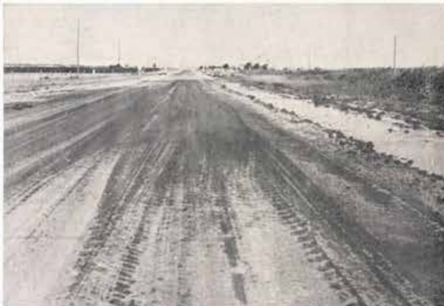
This silt covered portion on U. S. Highway 86 in Parmer County was the site of a serious wreck. A pickup truck overturned when it ran into the silt that had been deposited on the road by tailwater escaping from a neighboring farm. Could you be creating such a hazard by letting water escape from your land?
