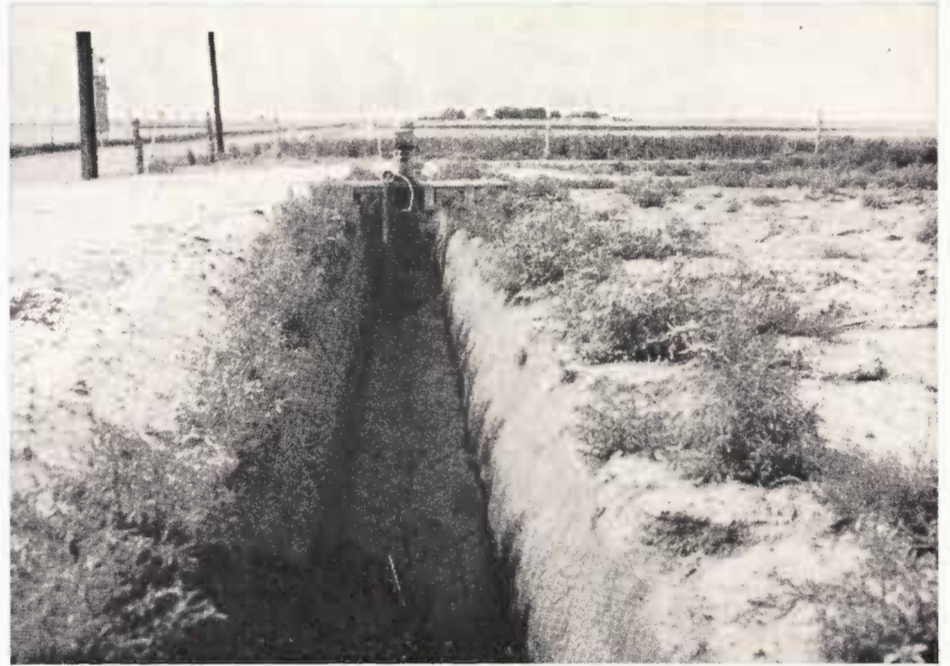
The above picture shows the tailwater ditch and pump assembly. Notice the silt in the bottom of the ditch. Some of this silt came from the sides of the ditch as they caved off some loose soil.
