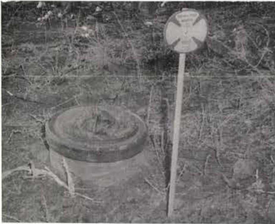
Shown here is the placement of a Break-Over Marker before the land is worked. The disc at the top of the device is rubber to prevent tools from hanging as implements are driven over the marker.
