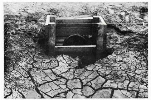
odd looking structure is simple but effective. The wooden box surrounds the intake pipe of a tailwater pit. By adding sections to the front of the box, water is dammed up and allows the silt to settle out of the water before it enters the pit.
