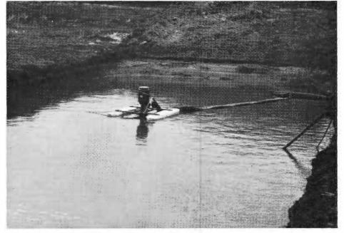
Extensive use of tail water pits in the High Plains Water District has brought about many new pumping installations. Illustrated is a new pump that floats on pontoons and rises or descends with the level of the water in the pit.
