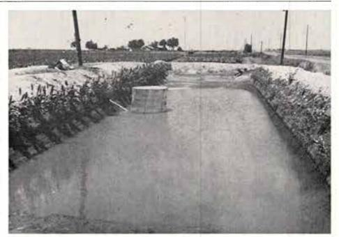
Delton Jack of Lockney uses this return system to capture 98 percent of his irrigation runoff. This system is in its second year of operation.
