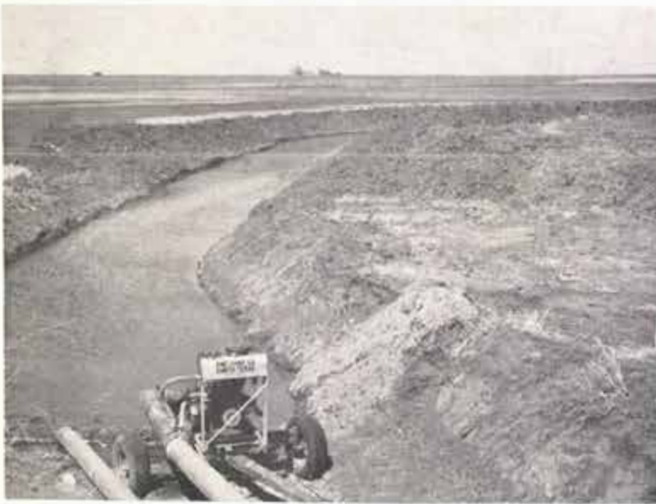
Playa lakes are being modified all over the High Plains. A simple modification shown here is channeling the water from the shallow parts of the lake to the pump. The lake water is pumped directly into a concrete line for distribution to crops.
