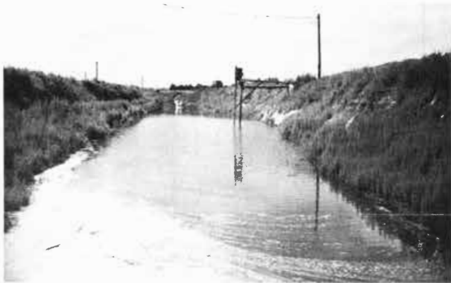
CURTIS TAILWATER PIT
