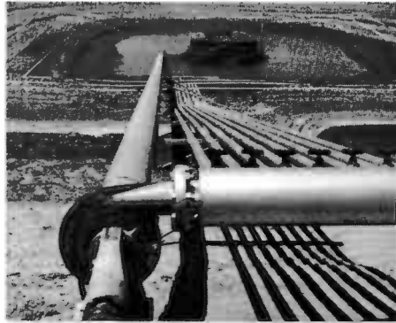
The centrifugal pump and the silt suspension return flow pipe layout in the Schlabs tailwater return pit. The square pattern of the silt suspension pipes can be seen in this photograph. These are 2-inch plastic pipes with 1/4-inch holes, four feet on centers, drilled in the top.
