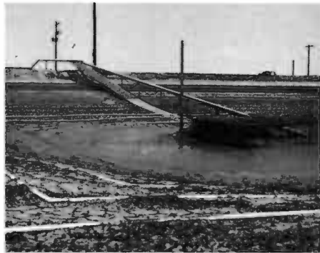
The screened structure in the center of the Schlabs pit (right center of this photograph) surrounds the inlet pipe to the pit. The stake to the left of the screened inlet is a staff gage from which the depth of the water in the pit can be read. The centrifugal pump is controlled by a switch that in turn is activated by the depth of the water in the pit.
