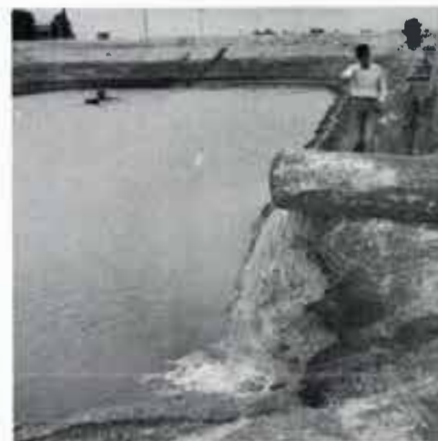
Raymond Rucker and Chester Mitchell discuss the clarity of the water that is entering the tailwater pit from the settling basin.
