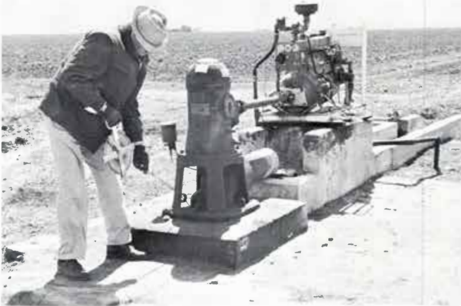
Inserting steel tape in well.
