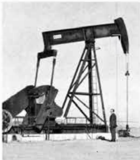
Long-stroke Getty Oil Company pumping unit on the Jones farm.
