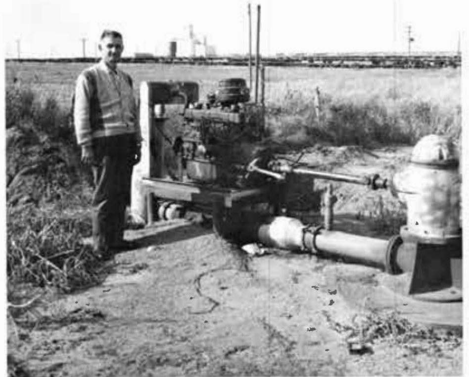
Cliff Thompson, a long time staff member of the High Plains Underground Water Conservation District No. 1 stands near an irrigation well being supplied natural gas as the energy source for its engine. Irrigation wells such as these have permitted the growth of the highly stable economy which exists on the High Plains. In the background can be seen a large cattle feed lot. The growth of this new industry in the High Plains has been a result of the consistently high yields of grains due to irrigation.
