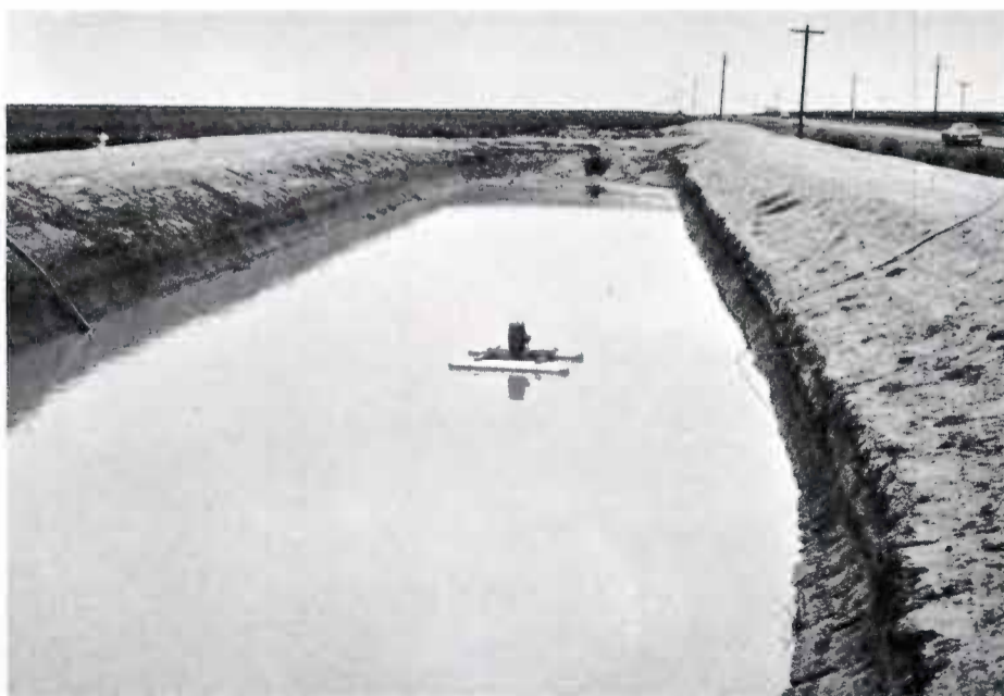
Shown is a newly constructed tailwater return system in Parmer County. Tailwater pits of this type have proven to be a very good means of conserving ground water.
