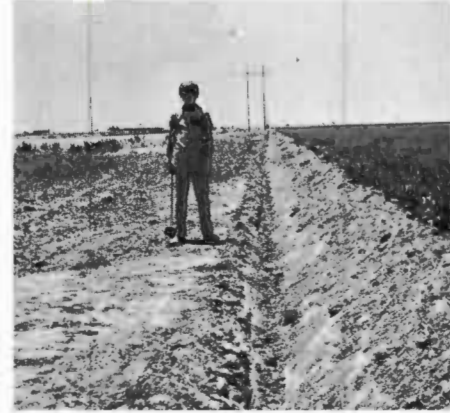
Most irrigation farmers do not set aside enough of their fields to provide adequate borrow areas for border construction and maintenance. Many of the borrow areas, and even some of the borders, extend onto public lands, as in the four pictures above and below.
