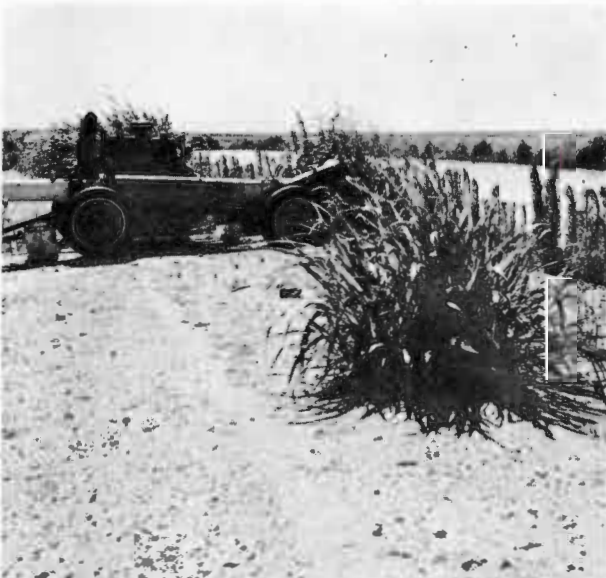
In the photo to the left is the engine that pumps 1,000 gallons per minute and irrigates six acres every 12 hours. The middle frame pictures a two-acre-foot settling pond Vise designed to trap silt before it enters the four-acre-foot pit. In
