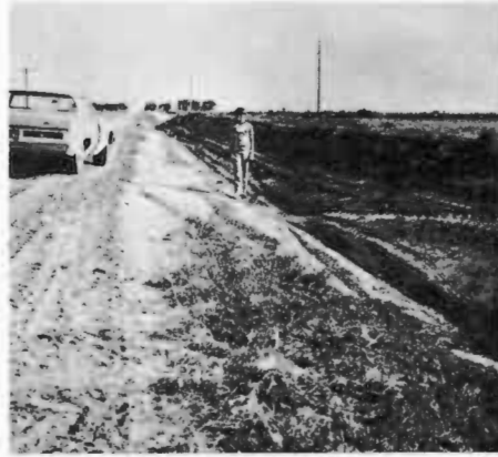
Most irrigation farmers do not set aside enough of their fields to provide adequate borrow areas for border construction and maintenance. Many of the borrow areas, and even some of the borders, extend onto public lands, as in the four pictures above and below.
