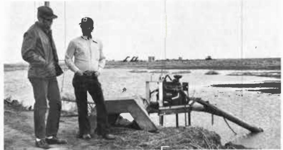
Pictured above is the modified playa lake on Schlabs' farm. The lake can hold 30 acre-feet of water at capacity.
