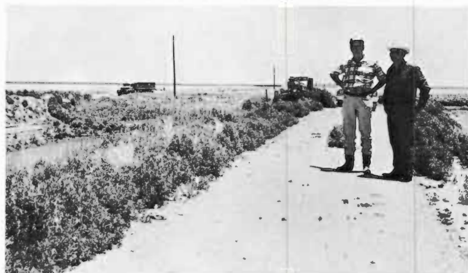
Reznik and Obbie Goolsby, District Field Representative, are shown standing beside Reznik's newest tailwater pit, dug in 1968. Reznik has the tailwater tied, with his five wells, into his entire irrigation system. He says a tailwater pit equals the same irrigation capacity as one eight-inch well.
