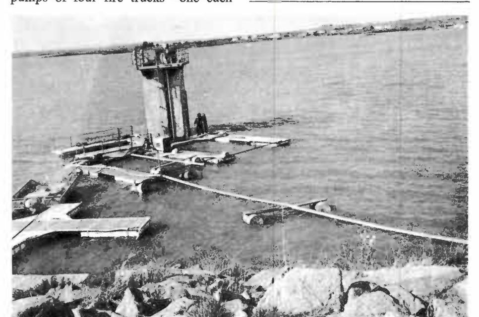
Deep-sea divers (to right of intake tower) and dredge pump used to remove silt and repair the White River Lake intake structure.
