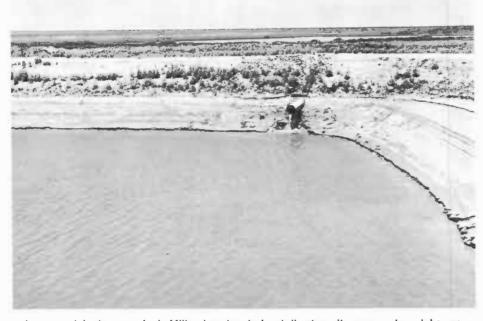
In several instances, Jack Miller has located a tailwater pit near a playa lake, so that the playa can serve as a settling pond (by itself, or in conjunction with a small silt pit) to trap silt before it enters the tailwater pit and clogs the lake pump. Note the lake in the background at the top of the photograph.
