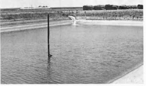
Shown here is one of the methods utilized on the Miller farms whereby water caught at other locations flows into a tailwater pit, where it remains until it is pumped into an underground pipeline system and back on the land for irrigation of more than 2,000 acres of beets, corn, milo, cotton and alfalfa.
