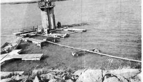
Deep-sea divers (to right of intake tower) and dredge pump used to remove silt and repair the White River Lake intake structure.
