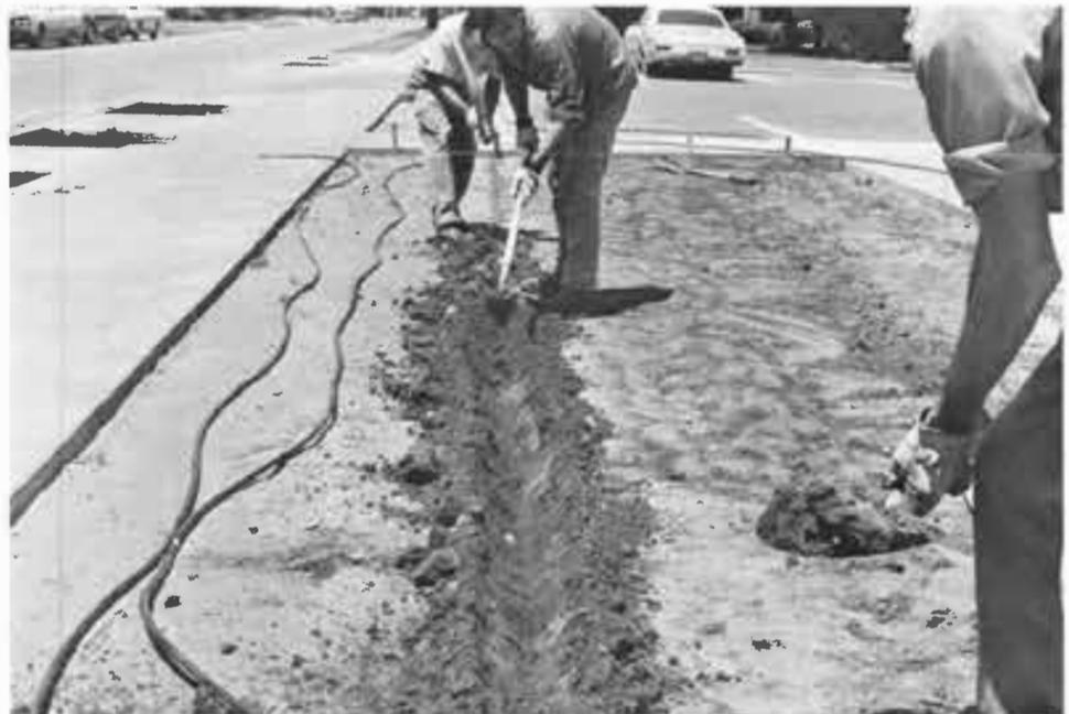
DIGGING DITCH AND LAYING EMITTER TUBING
