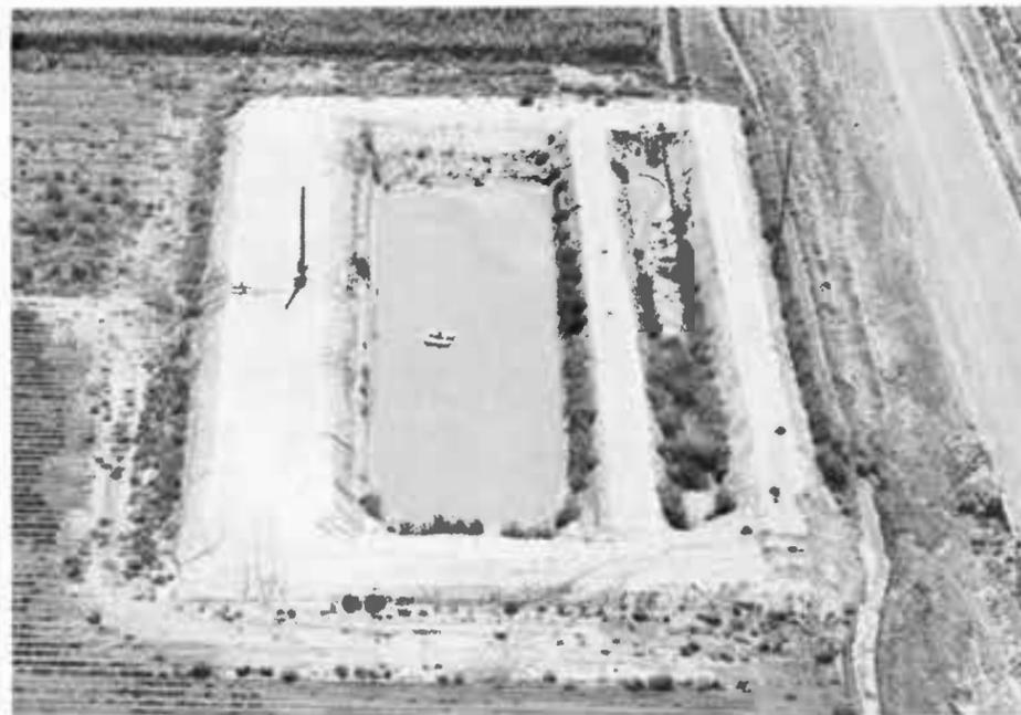
This tailwater pit captures runoff irrigation water, keeping it from escaping into the bar ditch, and recirculates it back over the land for other irrigations, thus, saving energy, groundwater and money. (District Photograph)
