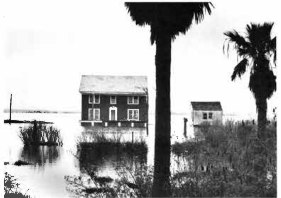
The home pictured above, once part of the Brownwood Subdivision, Baytown, Texas, is now permanently abandoned because of rising tidewater. This problem, caused by land surface subsidence, has led to the creation of the Harris-Galveston Coastal Subsidence District, the primary purpose of which is to "end subsidence".
