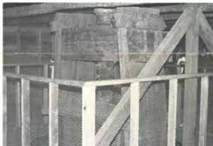
(3) Ground-level view of the wooden screw press which was powered by two mules, (4) Second floor view of the screw press.
