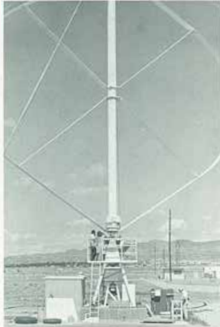
A wind turbine at the Sandia Laboratories in Albuquerque bears little resemblance to the eclipse windmill which dotted the High Plains of Texas in years past. The new-style windmill is being studied as an alternative source of energy and can produce 60 kilowatts of electricity in a 30-mile-an-hour wind. The windmill is a research project funded by the Energy Research and Development Administration (ERDA).
