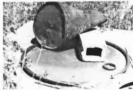
OPEN OR IMPROPERLY CAPPED WELLS are potential death traps. District rules require owners to permanently cap open wells with a cover capable of sustaining a weight of at least 400 pounds.
