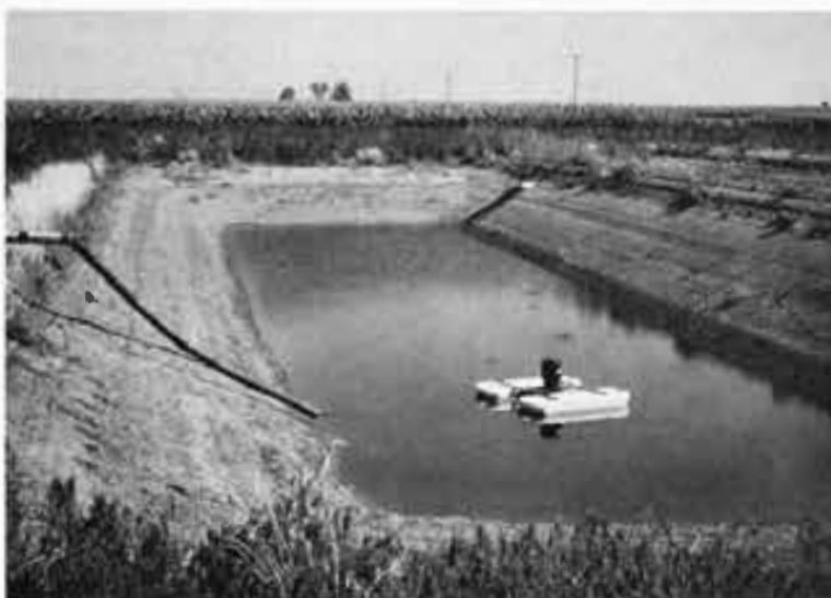
TAILWATER RECOVERY ponds and lake pumps capture irrigation runoff for reuse.
