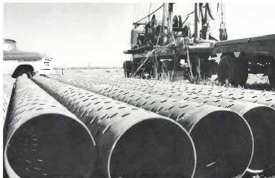
THE FIRST RECHARGE WELL drilled by the Water District was located at the Allmon Gin near Petersburg in 1955. Slotted casing was set in the well and playa water was recharged into it. Silt eventually clogged the formation.
