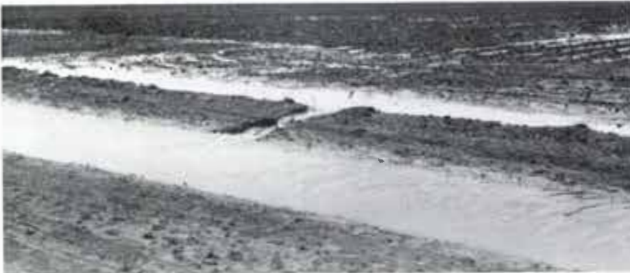
COUNTY ROAD BAR DITCHES may hold tailwater waste from furrow irrigated fields, but using the ditches for this purpose is a violation of the law.
