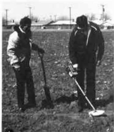
**DETECTIVE WORK**—Metal detectors are used to locate the buried neutron access tubes. Once located, the tubes are uncovered for readings.
