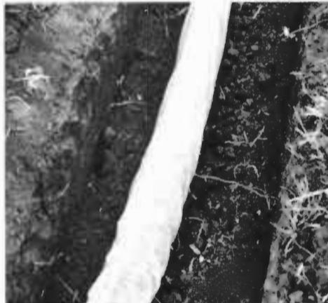
**FILTERS IN PLACE**—Sixteen-inch wide and 16-inch deep V-shaped trenches were dug in the base of the playa. A geotextile fabric filter was then slipped over three-inch diameter flexible plastic pipe like a sleeve. The fabric-covered pipe was then laid in a gravel bed in each trench, and six inches of sand and six inches of natural playa material backfilled each trench.
