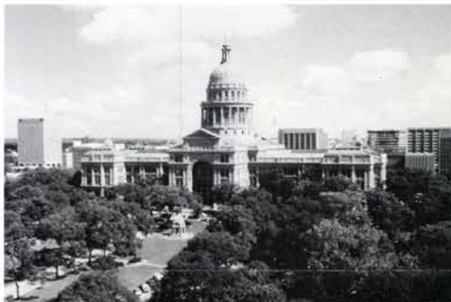
STATE HOUSE —The State capitol building in Austin (above) was the site of numerous discussions concerning the protection and management of ground water during the recent 70th Texas legislative session. Nearly 50 water-related bills were introduced by lawmakers during this time.
