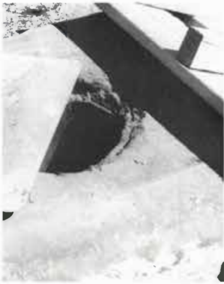
HAZARD — Dangerous open holes, as shown in this file photo, may be found dotting the South Plains. Producers should check all abandoned well sites on their property to make sure the well is properly capped.
