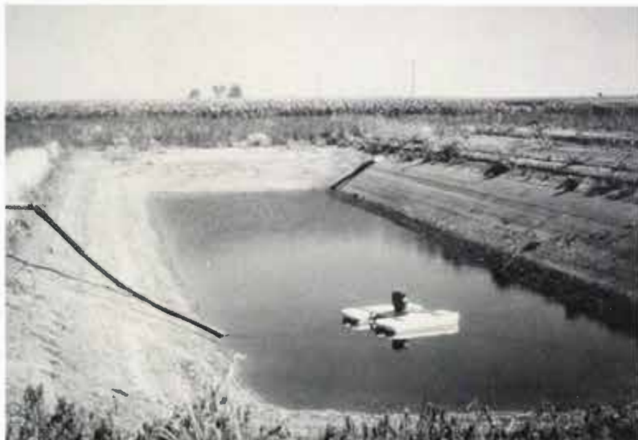
TAILWATER PITS COLLECT RUNOFF FOR LATER USE — By capturing runoff from the field and making it available for re-use, tailwater pits reduce the amount of water irrigators must pump from the Ogallala Aquifer. More than 3,000 tailwater return pits are currently in use within the High Plains Water District service area.
