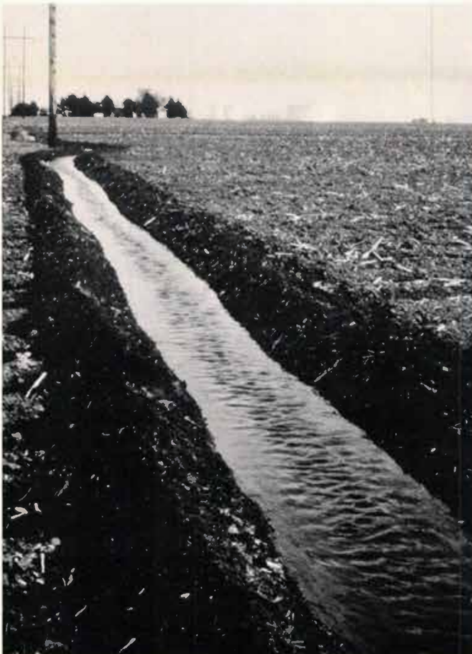
OPEN DITCH WATER LOSSES — Deep percolation and evaporation from open, unlined ditches result in water losses of 10 to 30 percent per 1,000 feet of ditch. The total water loss per foot of ditch in a 2,000 hour irrigation season averages about 5,000 gallons of water.
