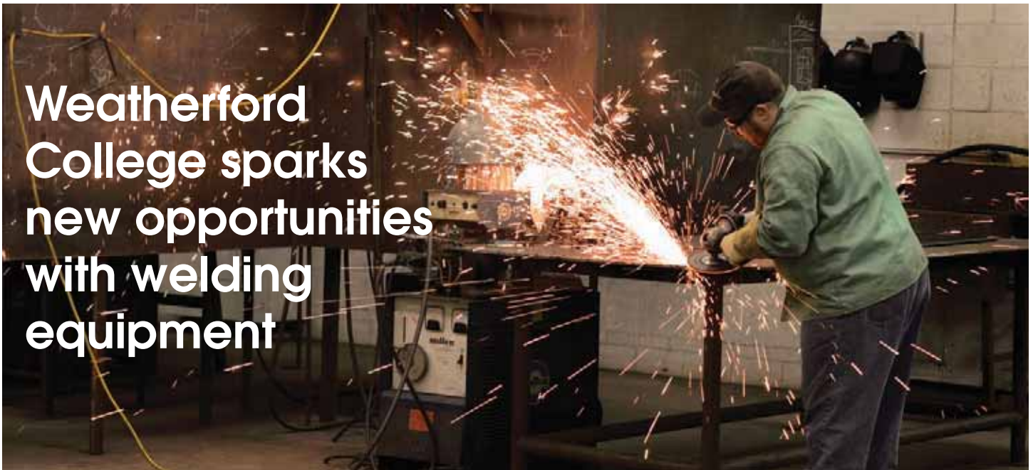
Weatherford College welding student Clay Youngblood works on obtaining his Basic Welding Technology Certification. Photo courtesy of Weatherford College
