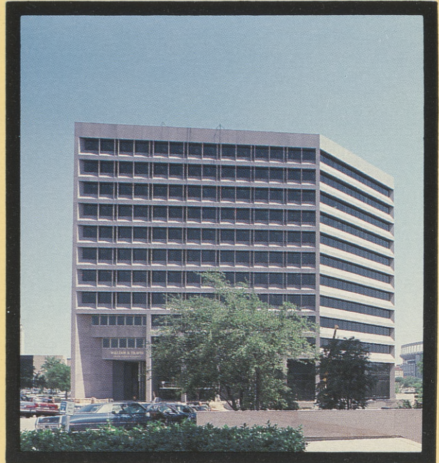
WILLIAM B. TRAVIS BUILDING
