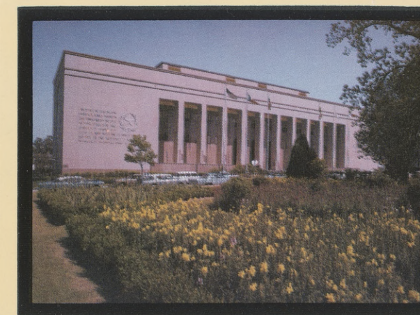
LORENZO DE ZAVALA STATE ARCHIVES AND LIBRARY BUILDING
