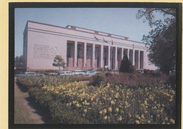
LORENZO DE ZAVALA STATE ARCHIVES AND LIBRARY BUILDING
